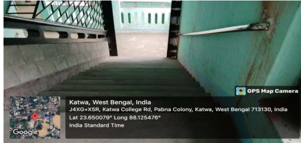
Installation of hand Railings in the staircases
