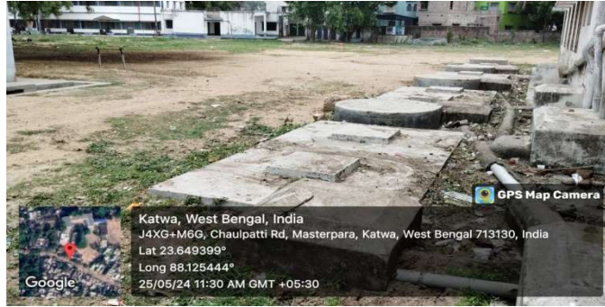
Waste water recycling through soak pit
